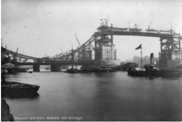
Picture 9 – Building a bridge.
