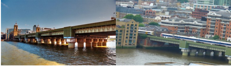
Picture 13 – Cannon Street Railway Bridge
