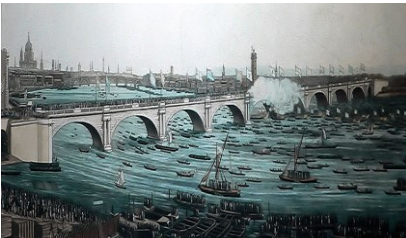
Picture 5 – Waterloo Bridge, June, 1817
