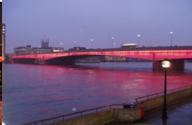
Picture 4 – Bridge lights at night
